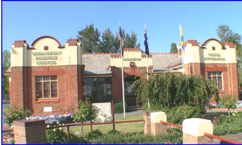
QBC and VIC HQ is located in the heart of Queanbeyan at the former QCC Council Chambers, 1 Farrer Place.
